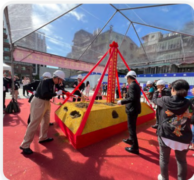
Groundbreaking Session (Huancui Section Project)
