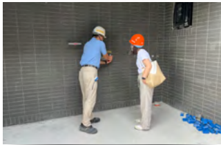
Indoor Water Pipe Pressure Test Tour
