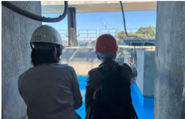
Top right image: Indoor water pipe pressure testing visit (Ruentex Fuyang) Bottom right image: Penthouse roof waterproofing testing visit (Ruentex Fuyang)
