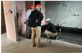
Bathroom and Kitchen Waterproofing Water Testing Visits
